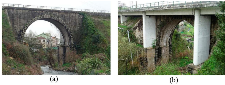
Figure 1. Leça railway bridge: (a) upstream view, and (b) downstream view.
