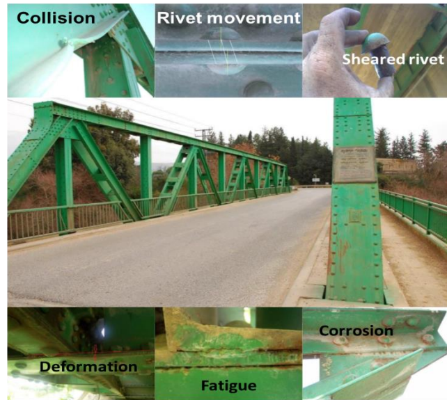
Figure 7. Steel truss bridge, Israel.
