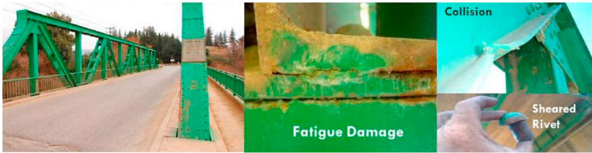
Fig. 7. Steel truss bridge, Israel.
