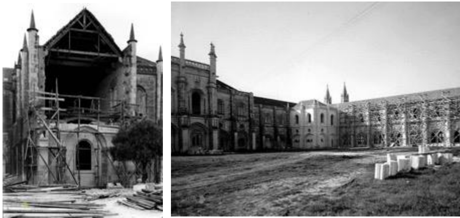
Figure 8: left: Photograph of the construction of the facade at the end of the aborted east wing, c. 1939, Foto 00503331, © IHRU/SIPA; right: West wing mid-construction and new staircase outbuilding, 1961, Foto 00503653, © IHRU/SIPA.
