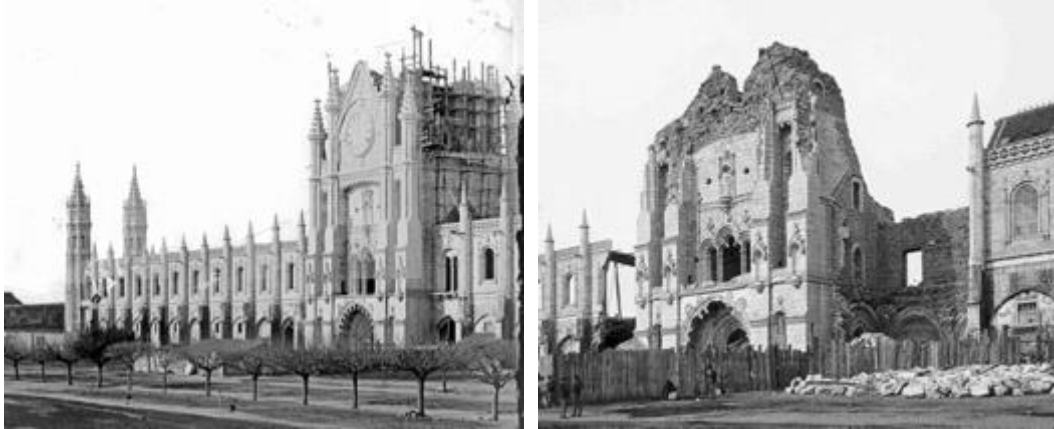
Figure 5: left: Photograph captured during the construction of the central tower, unknown author, 1877, © Arquivo Municipal de Lisboa; right: Photograph captured after the collapse of the central tower, Henrique Nunes, 1878, © Arquivo Municipal de Lisboa.
