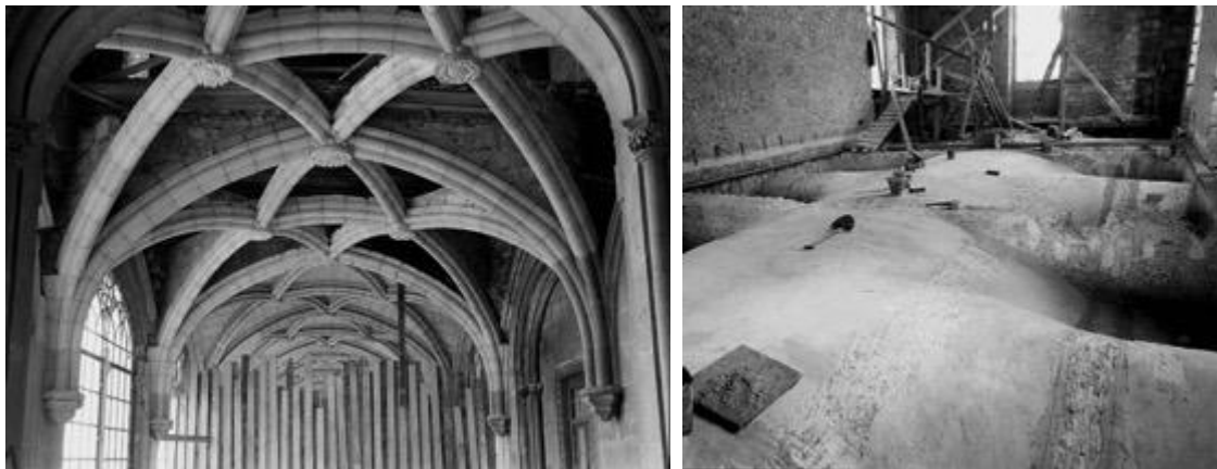
Figure 9: left: photograph of the gallery vaults under reconstruction next to the central body, c. 1939, Foto 00502933, © IHRU/SIPA; right: photograph of the extrados of the east wing vault, c. 1939, Foto 00503336, © IHRU/SIPA.
