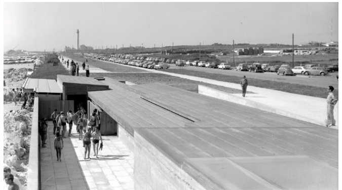
Figure 8 – Ocean Swimming Pool, building housing the changing rooms 1965. (Arquivo Câmara Municipal de Matosinhos)
