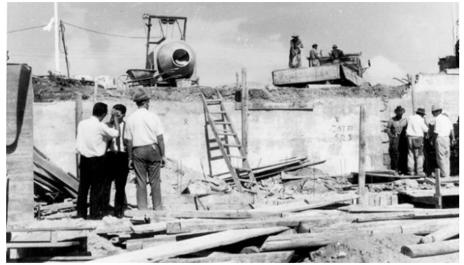
Figure 7 – Ocean Swimming Pool, construction of the southern area (Mota, 1872; Centro de Documentação da FAUP)
