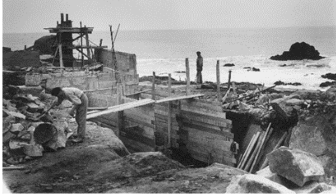
Figure 1 – Boa Nova Tea House and Restaurant, concrete foundations, 1959. (Câmara Municipal de Matosinhos)
