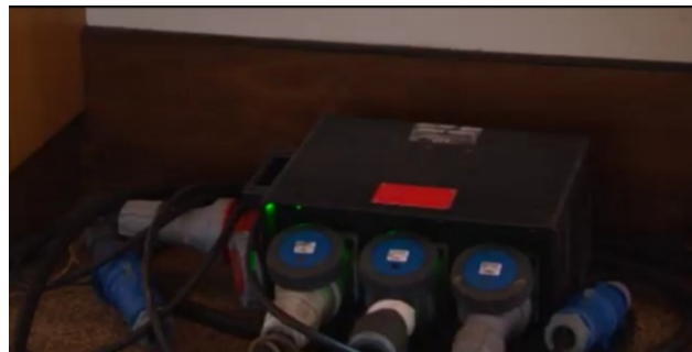
Figure 12: The three main cables. Source: Photo by the author, 2017
