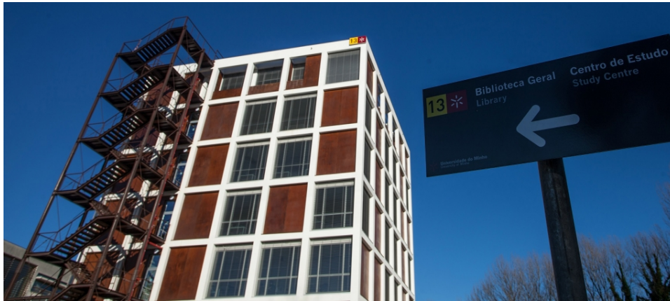
Figure 31 – UMinho library building in Guimarães (Mais Guimarães, 2018)
