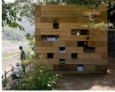
Fig.47. Wooden House, Sou Fujimoto.
