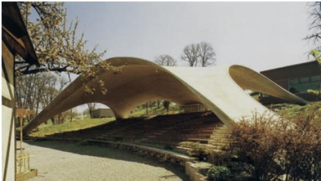
Figure 1 – Compression-only shell structure - Aichtal Outdoor Theatre in Germany (Adriaenssens et al. , 2014)
