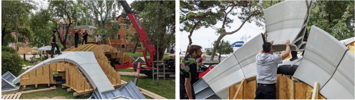
Figure 11 – The Striatu Bridge being built through the assembly of modules (Lomholt, 2021)
