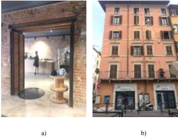
626 Figure 1. Example of new openings made at street-level of URM buildings in Brescia (Italy).
