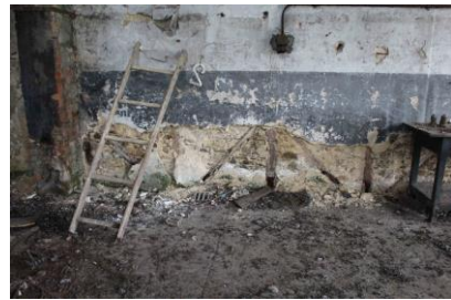
c) Diagonal bracing within a masonry wall
