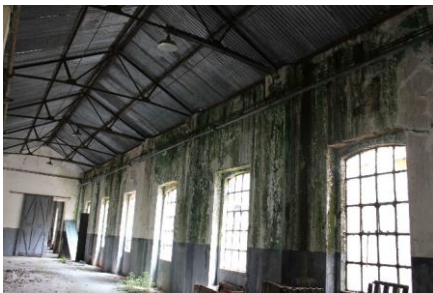
(d) Corrugated steel roof (a) left exposed in a workshop space
