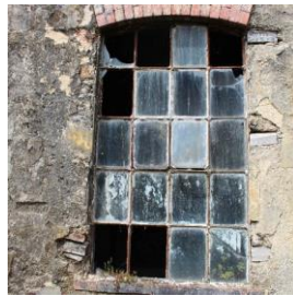
b) Timber inclusions concentrated around the window openings
