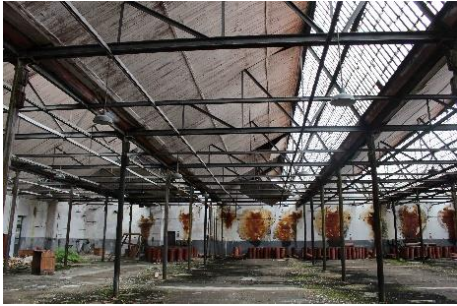
c) Room A (weaving section)
