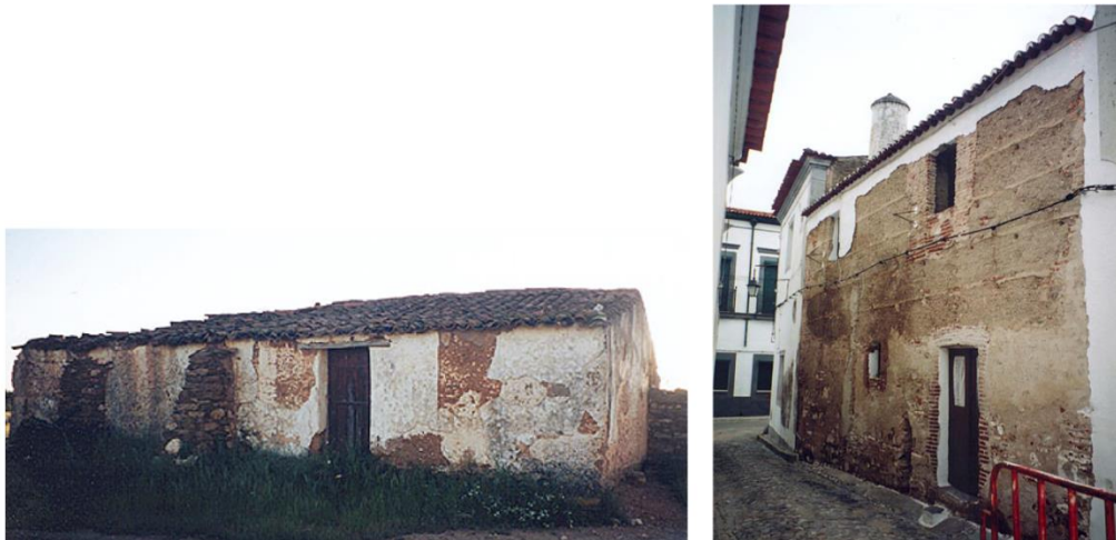
Figure 8. (left) Traditional rural one-floor rammed earth vernacular construction in Alentejo, Portugal (Correia 2007); and (right) Traditional urban two-floor rammed earth construction in Alentejo, Portugal (Correia 2002).
