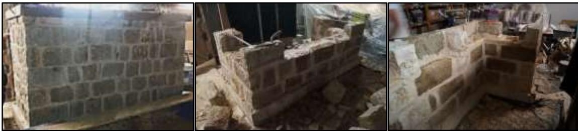
Figure 1. From left to right: WALL 0, WALL 1, WALL 2 construction phases
