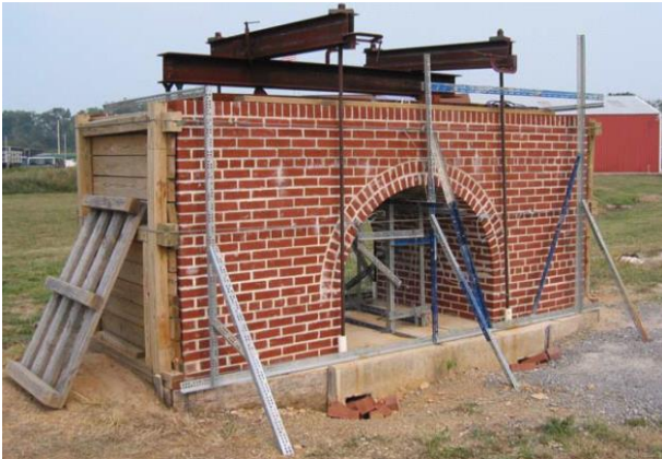
Figure 5. Large-scale bridge model
