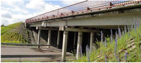
Figure 1. Side view of Assaku viaduct ( bms.teed.ee )
