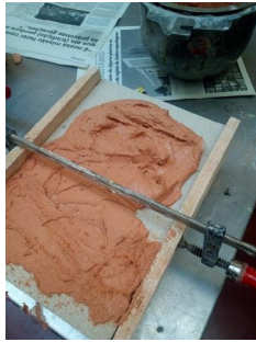
Laying the mortar on the support
