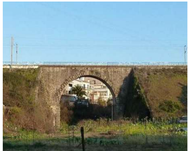
Figure 1. Leça railway bridge
