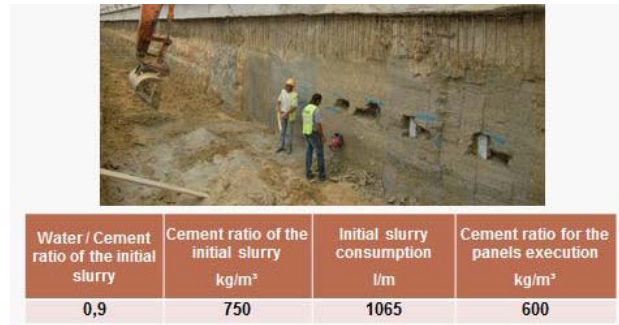
Figure 7. Adopted values for the CSM panels execution parameters.
