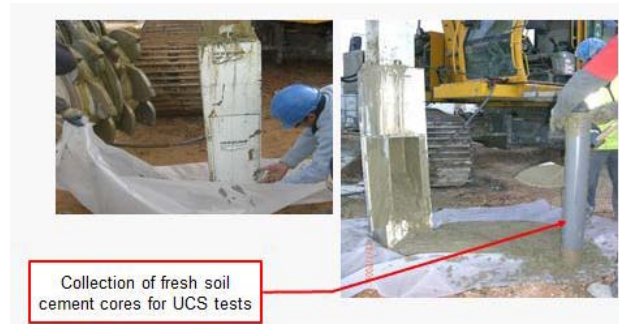
Figure 6. Collection of soil - cement fresh cores.
