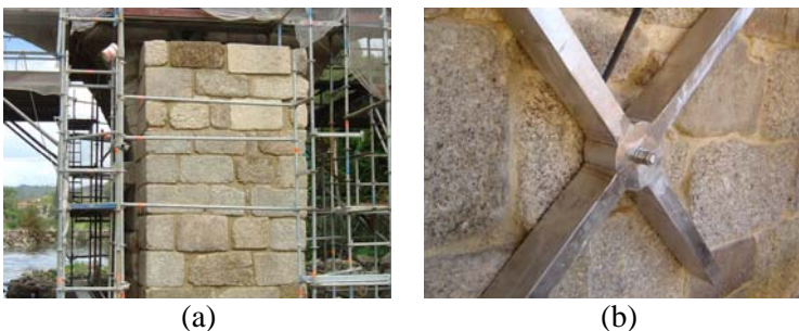
Figure 7. (a) Rebuilding of a downstream cutwater; (b) cross-shaped anchorage plate.
