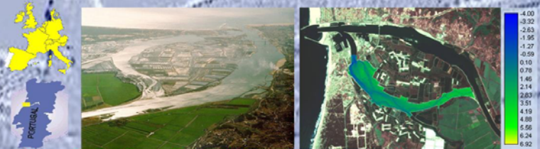
Figure 1 – Location, aerial view of Mondego estuary and south arm bathymetry
