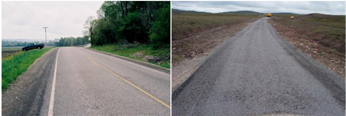
Figure 3. Completed construction: CR342, May 2004 after four years in service in New York State (left); B871 in Highland, UK, subject to heavy logging trucks (right, photograph courtesy Garry Smith, Highland Council)
