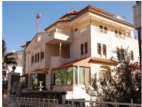
Figure 2.14 – Villa in Ramallah (Jordan Valley Witness, 2011)
