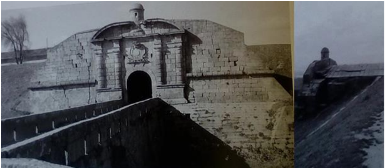
Figure 9. State of damage in the Gate of San Francisco year 1962
