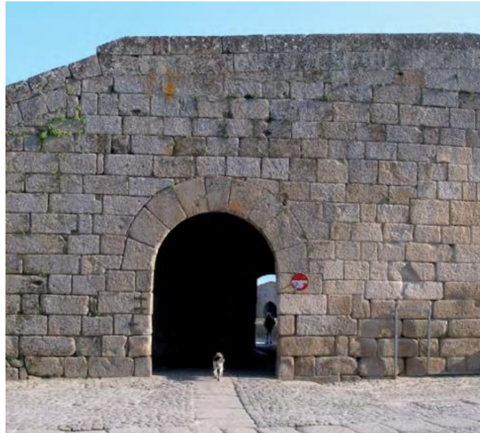
Figure 5. View from the interior of the Gate of San Francisco (Technical comission for the candidacy of Almeida, 2009)
