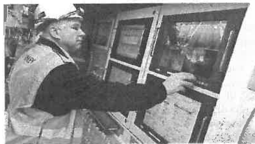
Figure 2. Boring head command centre (Crossrail, 2015).
