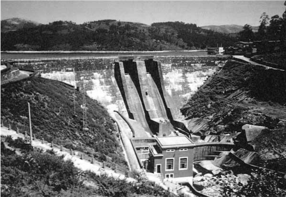
Figure 8 – View of Guilhofrei Dam from the downstream side
