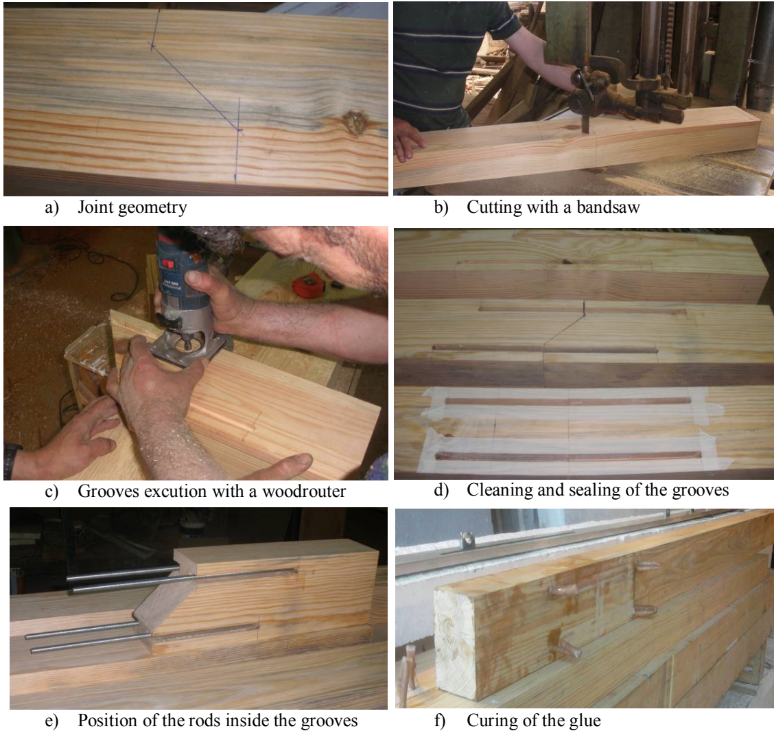
Figure 6. Main steps in the specimens repaired with timber prosthesis.
