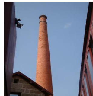
Figure 1. The masonry chimney.
