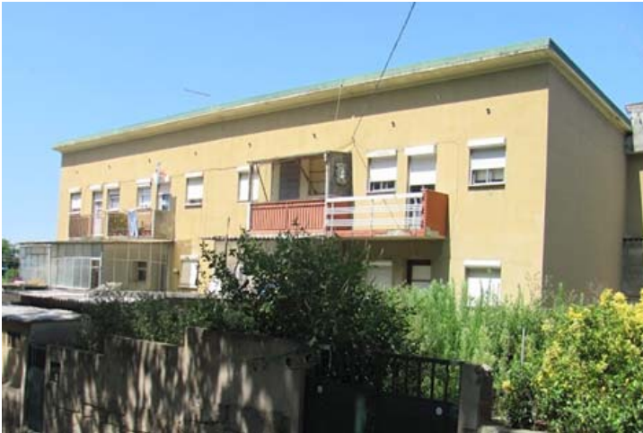
Figure 1: Building before renovation
