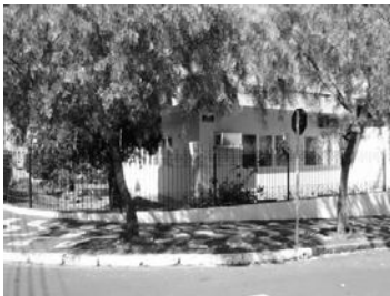
Figure 10. Windows of a building in Araras, which provide cross ventilation.
