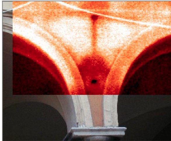
Figure 2.21: Detection of hidden tie rods using thermal vision [10]
