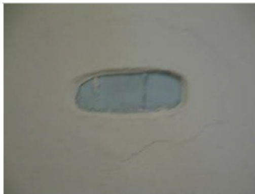
Figure 2.30: Glass pieces inserted into the wall to monitor cracks [2]
