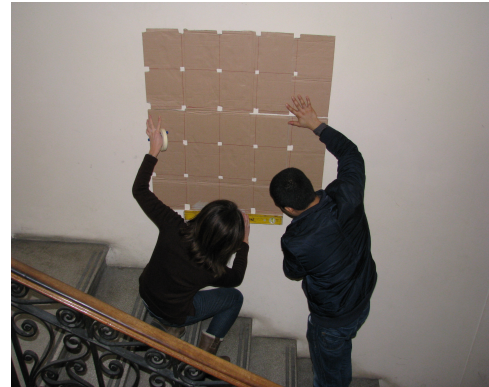
Figure 2.3: Installation of Grid for sonic test [2]
