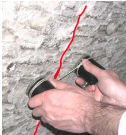
Figure 2.17: Performing Ultrasonic Test [10]
