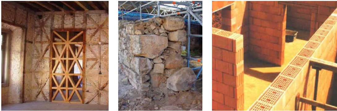
Figure 1. Examples of different masonry types (from left to right): timber braced “Pombalino” system after the 1755 earthquake in Lisbon; irregular stone wall with a complex transverse cross section; unreinforced masonry using blocks complying with thermal and sound regulations.
