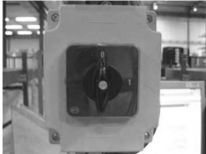
Figura 1 – Interruptor desligado
