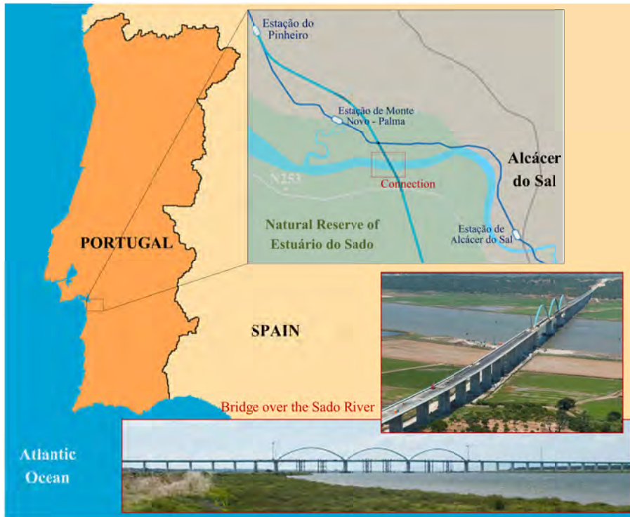
Figure 5.1 – Location of case study 2 (bridge)
