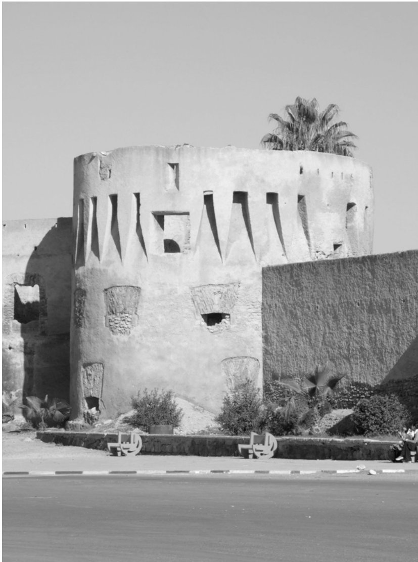
Fig. 6. Azemmour. Bastion of S. Cristóvão [St Christopher].
