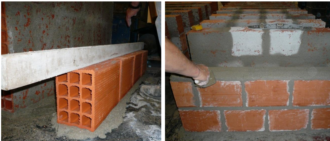
Figure 53. Construction of the walls. Leveling and control of bed joint thickness.
