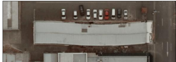
(b) Aerial view of building
