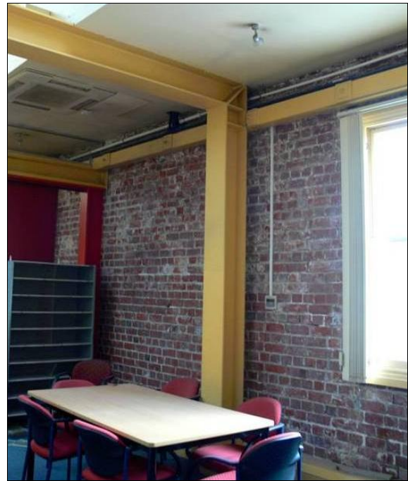
Figure 18: Internal view of steel moment frame retrofit.
