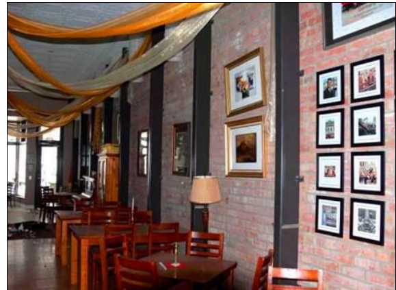
Figure 19: Steel strong-backs provided out-of-plane support for URM walls.
