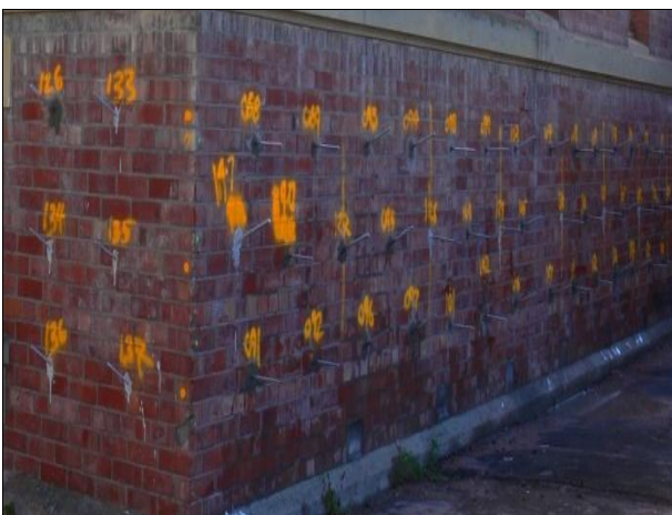
Figure 30: Typical test specimen arrangement.
