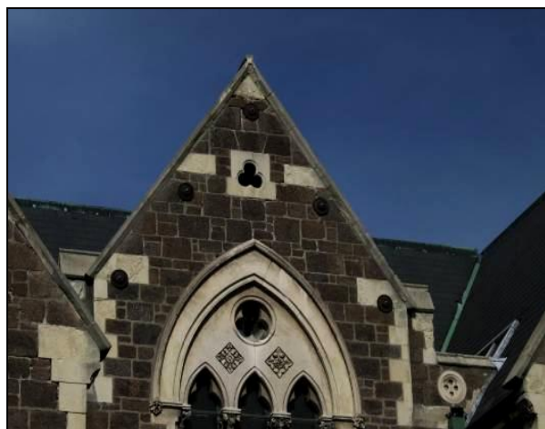
Figure 39: The Christchurch Arts Centre, showing successful use of wall-diaphragm anchorages.
