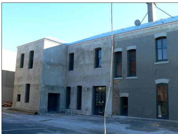
Figure 21: Rear of a building retrofitted using shotcrete.
