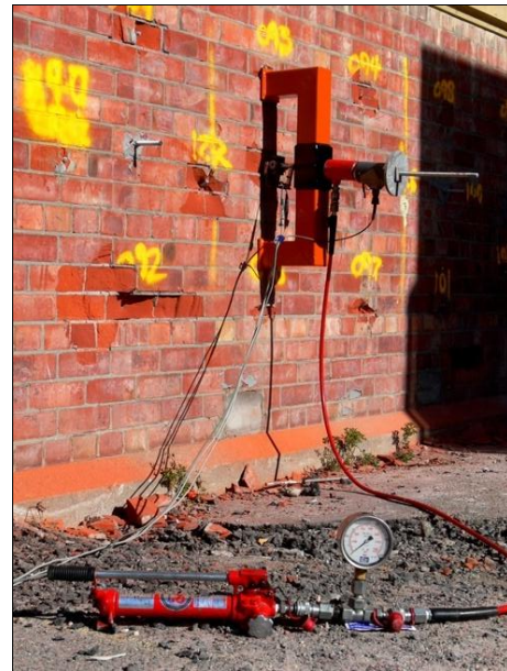
Figure 31: Typical test set-up used for pullout anchor testing.
