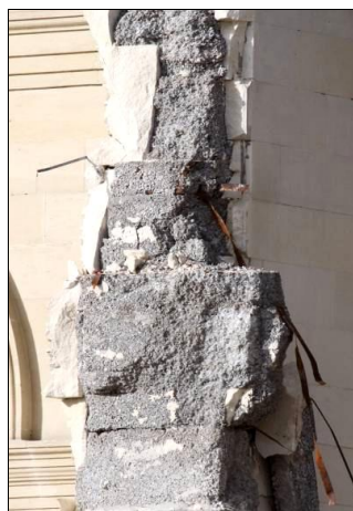
(b) Cathedral of the Blessed Sacrament - Oamaru stone with poured concrete
