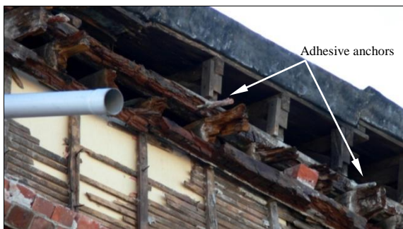
Figure 26: Adhesive anchors installed in a badly deteriorated roof diaphragm.
