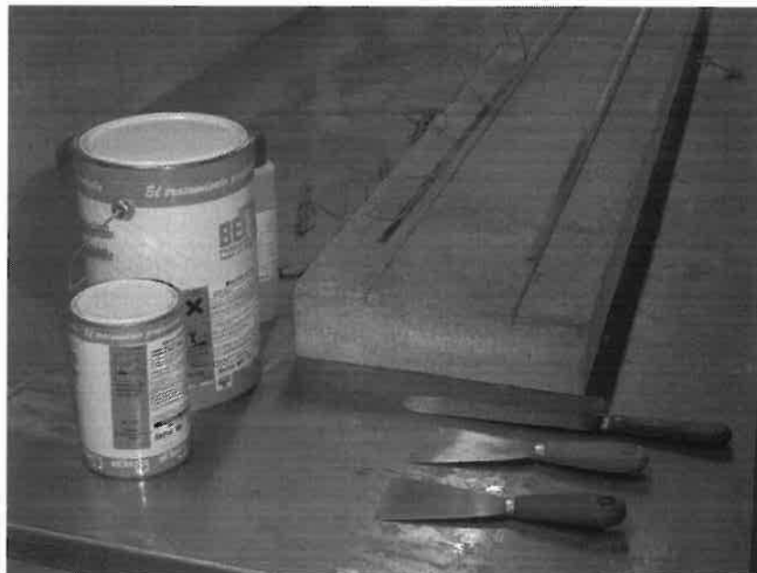
Figure 5.3 - A specimen before to be strengthened; the adhesive compound recipients; the acetone bottle; the CFRP laminate strips; and the tools used to mix and to apply the epoxy adhesive into the slits.
