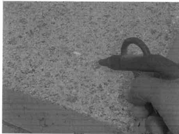
Figure 5.6 - Cleaning the sandblasted surface with compressed air jet.
