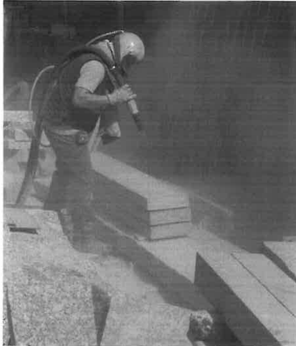
Figure 5.5 - Sandblasting the top surface specimen.
