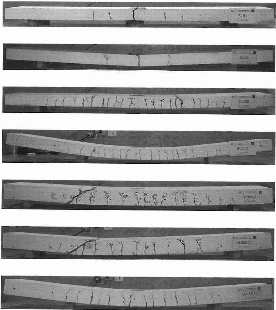
Figure G1 - Side view of the slabs after having been tested (the side view of the slab SL04S was not possible to be registered).
