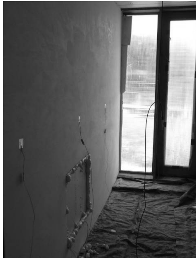
Figure 2: West room of the Passy's test cell – Gypsum-PCM façade.
