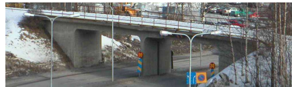
Figure 3: Örnköldsvik Bridge (Sweden)
