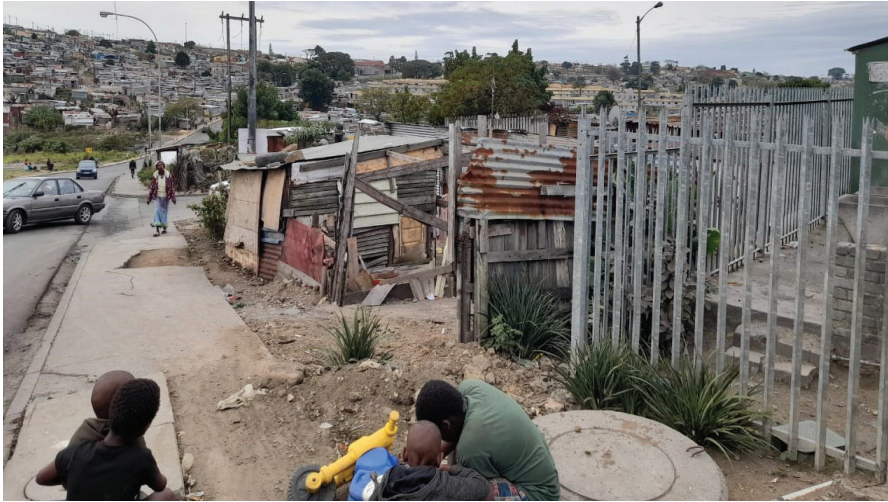
Figure 4. Street view of Duncan Village
