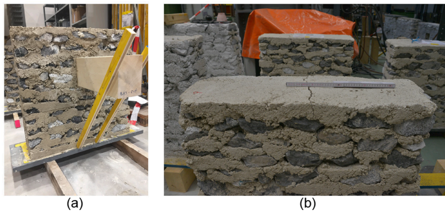
Fig. 3. PAT specimens: (a) construction; (b) existing crack (back view of the wall).
