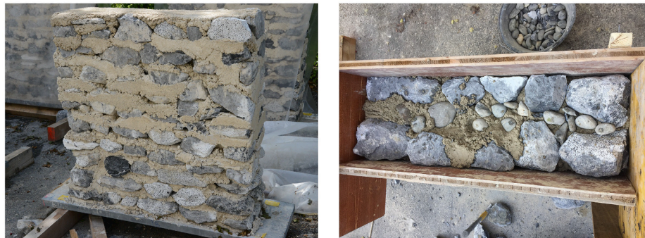
Fig. 2. Construction of the masonry walls.
