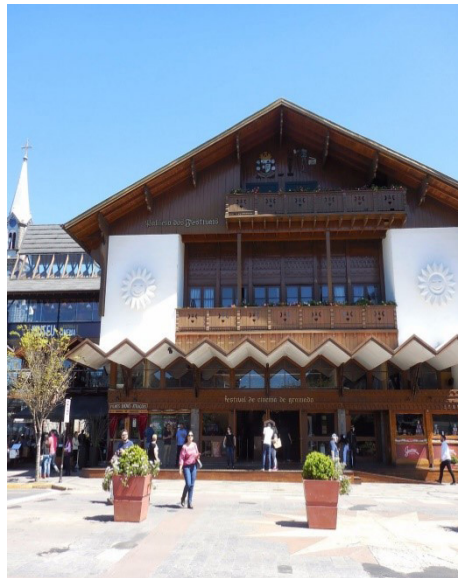
Figure 1. Palácio dos Festivais Building
