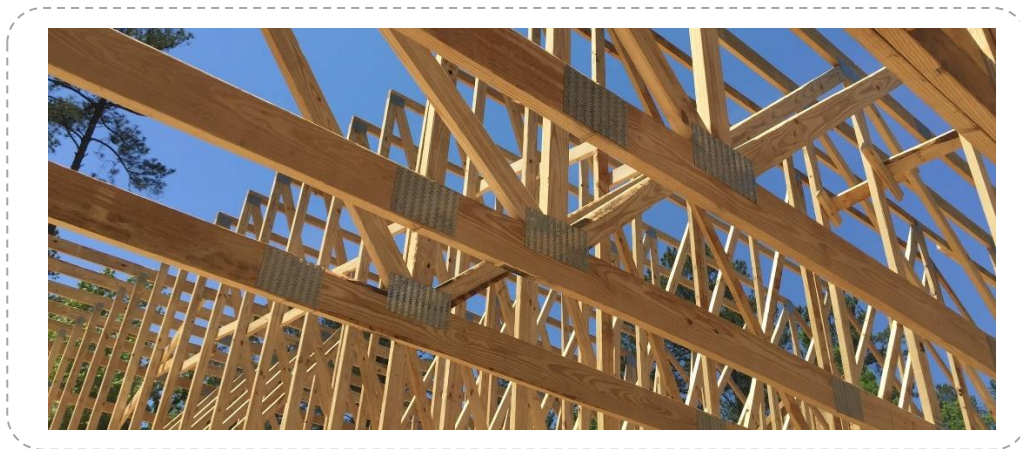
Figure 7: Component system construction. (Component Building Systems, Inc)
