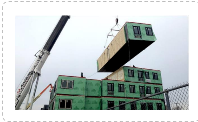
Figure 3 - Modular construction. (Modular Construction, Advantages and Challenges | Real Projectives)
