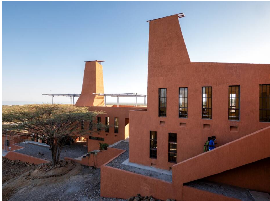
Figura 79 - Fachada Sul, Startup Lions Campus .
