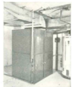
Carrier's unit includes gas heater.
