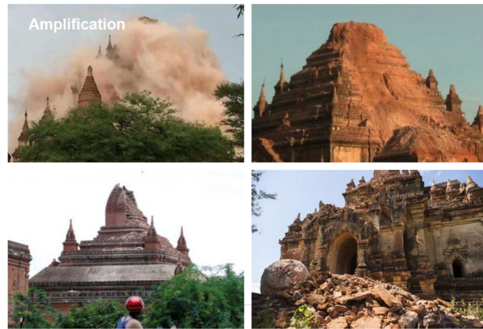
Figure 5. Amplification effects during the 2016 Bagan earthquake in Myanmar.
