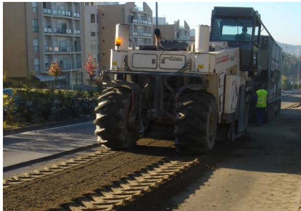
Figure 7. “In situ” recycling with cement on the trial section
