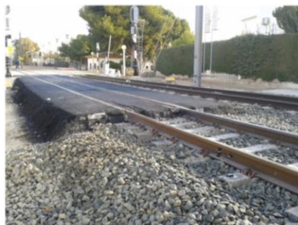
Figure 3.34 – Detail of the stretch of asphalt slab track (20 m) inserted between the previously existing concrete slab track and ballasted track (Real et al., 2016)
