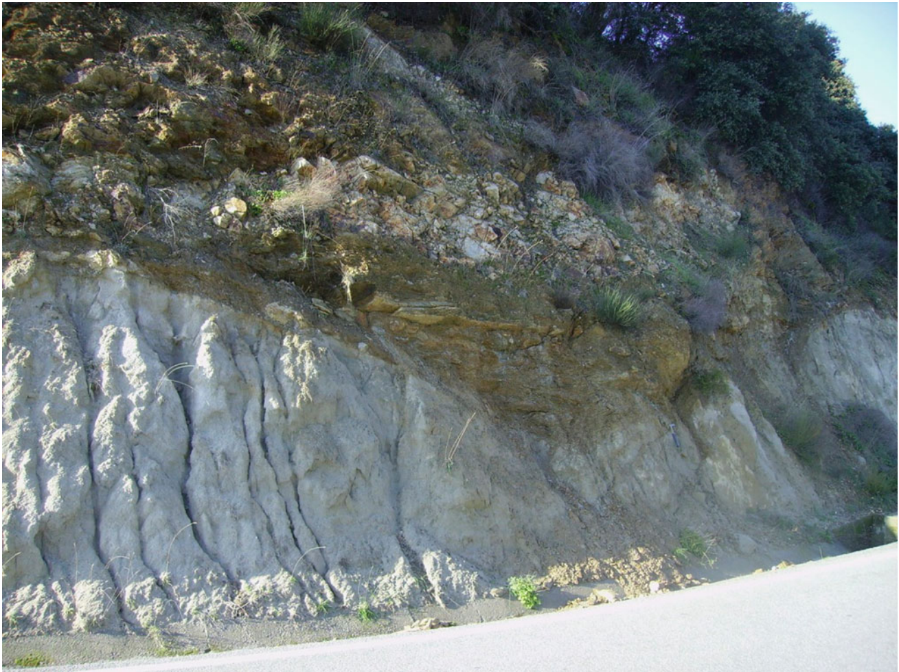
Fig. 11.7 Outcrop at the southern limit of the Longroiva basin documents the reverse movement of the Vilarica fault, with the Variscan bedrock (Cambrian) over the Vilarica Formation (Paleogene)
