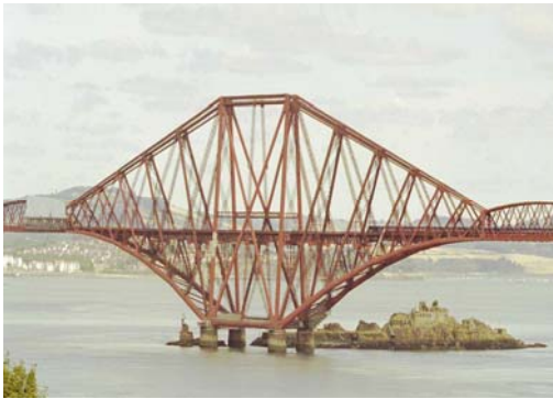
Figura 5.20 – Ponte Forth Firth
