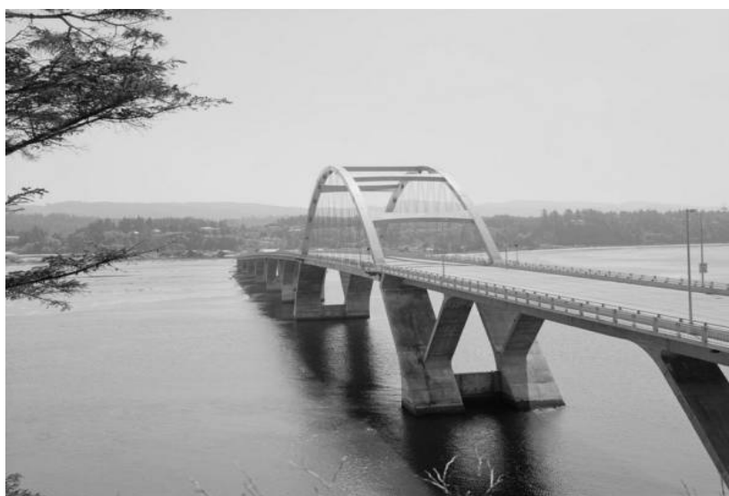
Figura 3.11 – Ponte “Alsea Bay”
