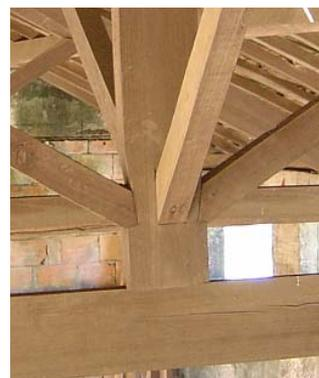
Fig 7 Example of a misconceived connection between the king post and the tie-beam
